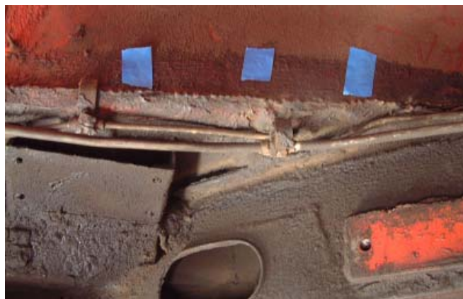
Fig 6 Here's a before shot from below of the transmission tunnel on the right side. Take note of the OEM sheetmetal tubing clips as they provide your best location guidance. Start by removing the fuel line and bending it towards the outside. Bend the clip in the same direction.
